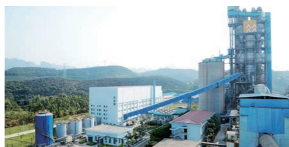
Tianyang Cement uses cement kilns to treat municipal solid waste.
