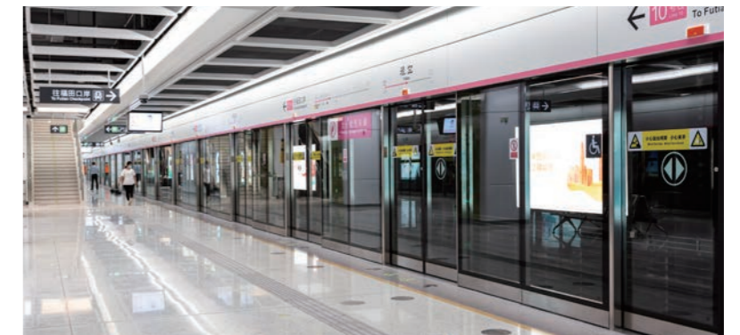
Construction of Shenzhen Metro Line 10 and Line 4 used 90,000 m 2 of inorganic engineered stones produced by CR Cement.
