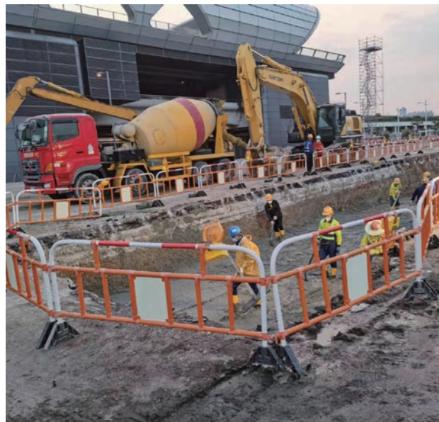
Construction site of the Fangcang hospital at Kai Tak Cruise Terminal
